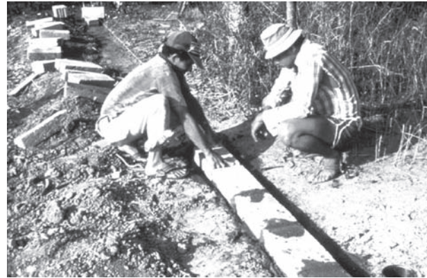
Figure 21-20. Laying down a foundation to support the external walls of a storeroom.
