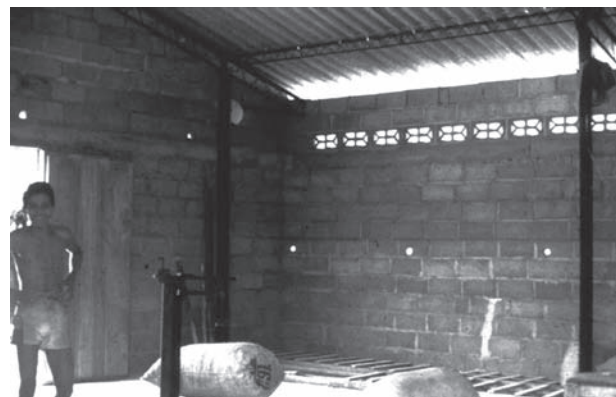
Figure 21-22. Wall with concrete fretwork running along its upper length.
